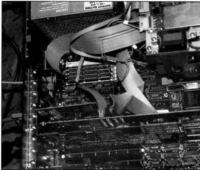
Figure 7. Installed in Computer.
