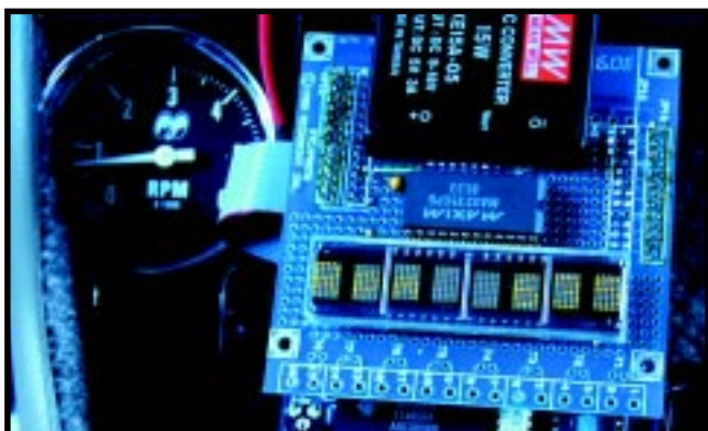
Photo 4—The old and new. Though seemingly analog, the dial gauges in the instrument panel are driven digitally. Even the radio is connected to the VCM, so the faster you go, the louder it gets.
