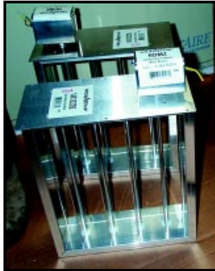
Photo 3 —Zone dampers use motors to slowly close the vanes inside the damper. When power is off, a spring opens the vanes. I may add leaf switches to ensure that the dampers close when powered. Right now, detecting problems is difficult because they remain open when off.
