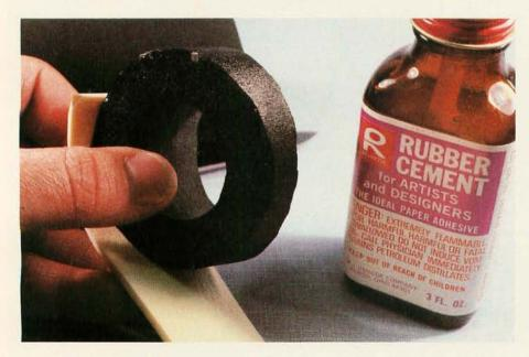
**Photo 5:** Adding pliable material to produce a tight fit around the phone handset. I found a plastic placemat at a discount store with a  $\frac{1}{4}$ -inch foam backing that was perfect. Cut a strip  $1\frac{1}{2}$  by 8 inches and glue this around the outside of the wedge as shown. Trim to the exact circumference and cover with a strip of fabric adhesive tape. The latter helps hold everything together.
