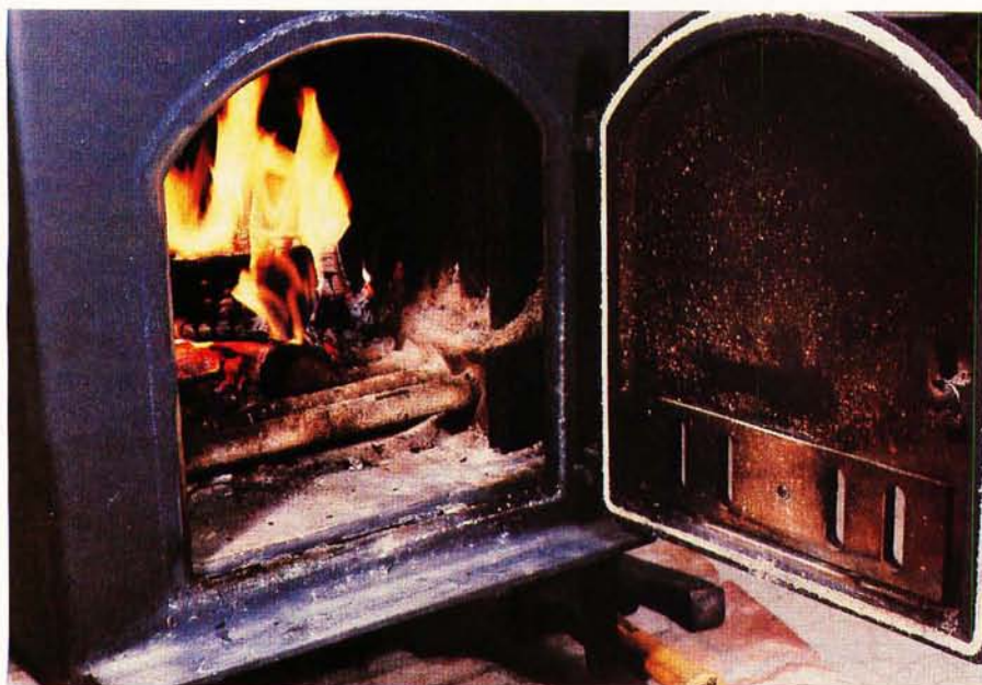
Photo 3: In operation, the heat from the fire warms the water in the tubes. This is a relatively small fire. The fire box is usually filled.
