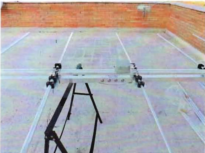
Ansicht Balunanschluss an Element S10 View of the balun mounted adjacent to element S10
